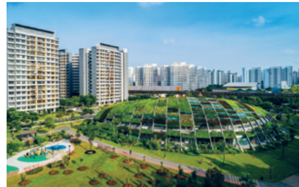
▲ A "rolling hill" façade helps the preschool blend in with the natural landscape. "The green roof provides a heat barrier for internal spaces, improving cross-ventilation and reducing air-con usage," say Freight Architects' directors, Mr Kee Jing Zhi and Mr Tan Kian Teck. They also worked with the centre and NParks to create a playground and community garden.
